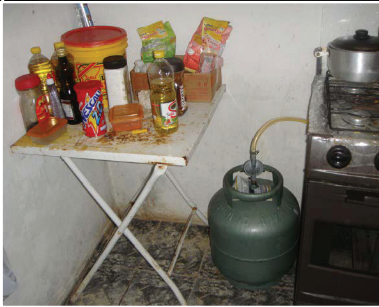
Gas cylinder kept in an inadequate place causing risk of an explosion and fire in the workplace.
